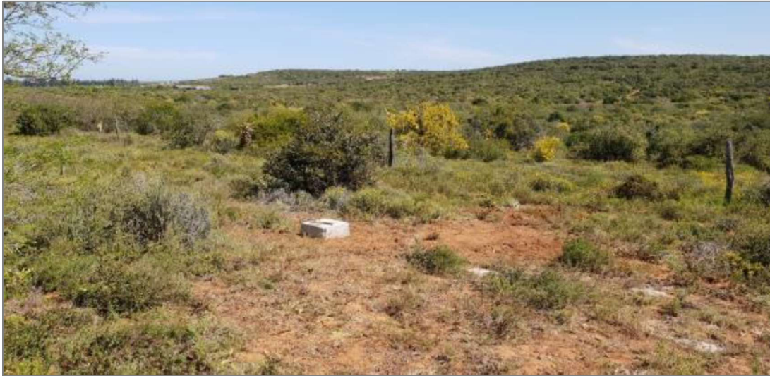
Plate 6-2: General view of left flank conditions, looking here along the spillway alignment in a downstream direction
